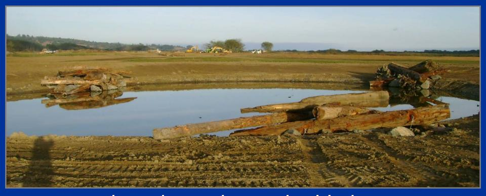
Logs Anchored together and cabled to 2-Ton Rocks. Each log required one 2-Ton Rock to counter buoyancy
