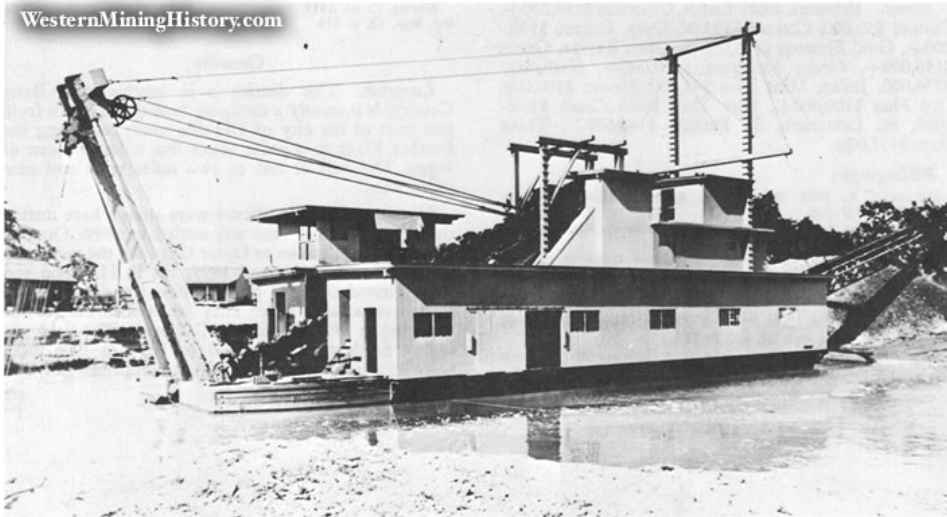
Photo 53. Cherokee Mining Company Dredge, Oroville District. This 1904 photo shows one of the earliest bucket-line dredges in California, operating here in Butte County.
