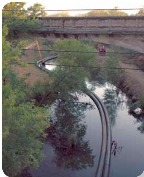
Side-by-side mile-long culverts being installed to move water from the upstream to the downstream extent of the Putah Creek channel project, summer 2011.
