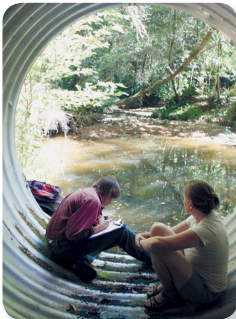
Geologist Bill Eastwood, Redwood Creek stream monitor, and Sara Schremmer, SRF, at a monitoring site where the summer flow trickles through a culvert designed for massive storm events. photo: Dana Stolzman
