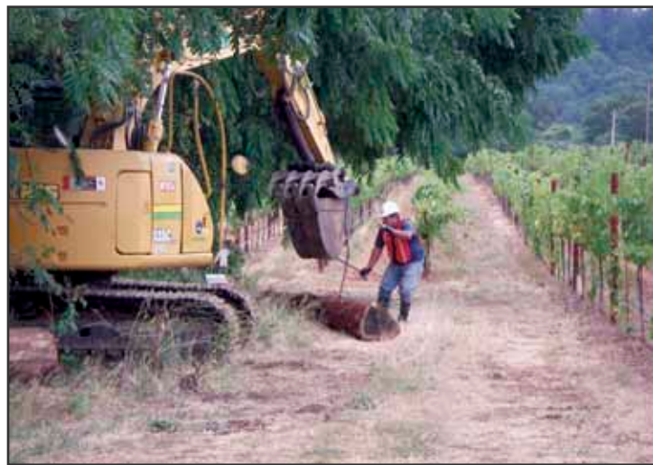
Grape Creek instream habitat improvement project in the Dry Creek watershed. Photo: Greg Fisher
