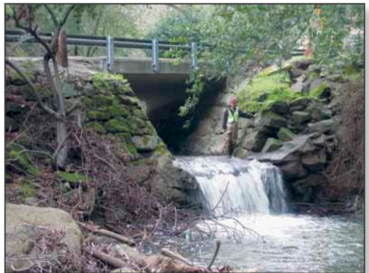
Historic culvert to be replaced on Stonybrook Creek as part of recovering steelhead in Alameda Creek watershed. Photo: Michael Love
