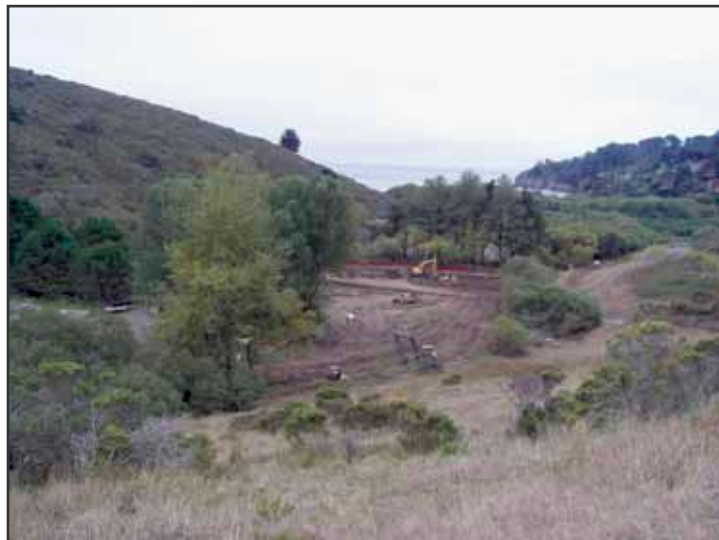
Construction at Green Gulch farm. Photo: Mike Jensen
