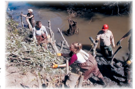
Constructing a bioengineering project on Freshwater Creek.
