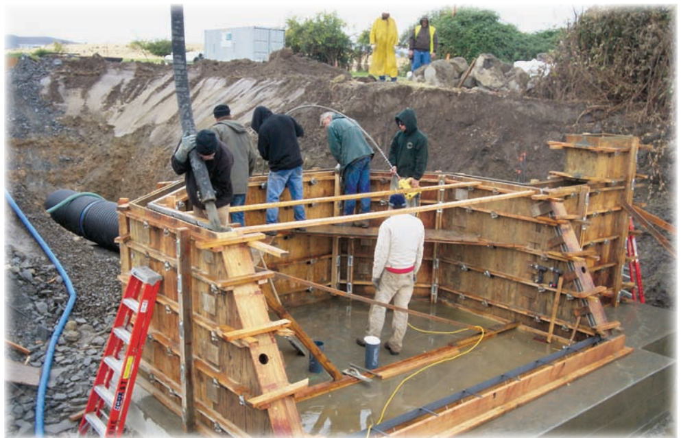
A Salmon barrier removal, fisheries enhancement, and agricultural water supply reliability project at Araujo Dam in Siskiyou County that was funded with IRWMP funds.
