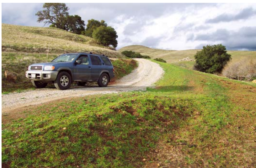
THE SAME ROAD OUTSLOPED WITH ROLLING DIPS
