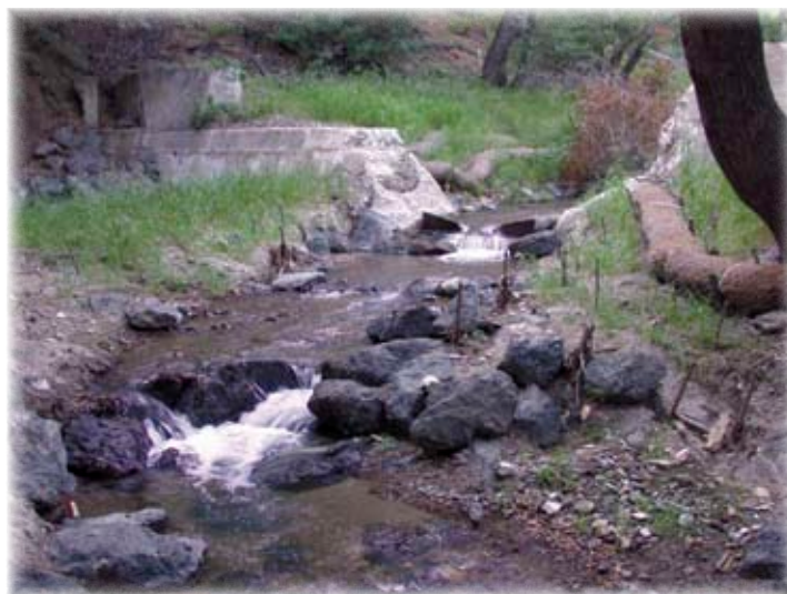
Dam removal upstream of Cuesta Grade in San Luis Obispo Creek
