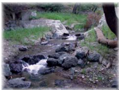
Grade control downstream of a fish passage project on San Luis Obispo Creek. The 14 ft water supply dam was partially removed. Stored sediments were excavated and used to fill the downstream channel to provide passage for steelhead.
