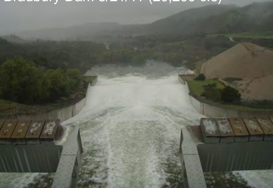
Bradbury Dam 3/21/11 (20,200 cfs)
