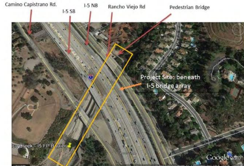
TRAFFIC STRUCTURES IN VICINITY OF I-5 CROSSING TRABUCO CREEK
