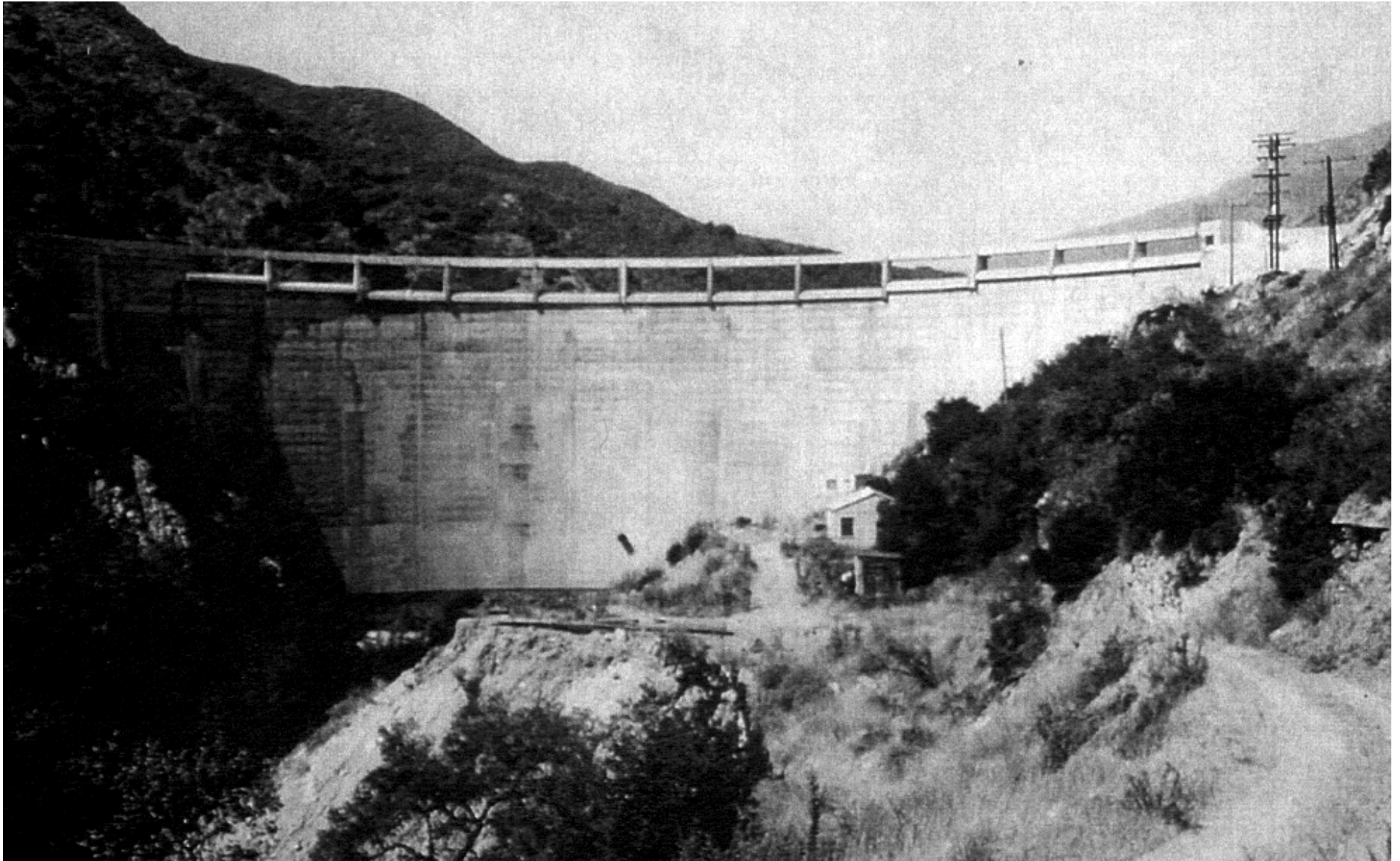
Matilija Dam as constructed 1948
