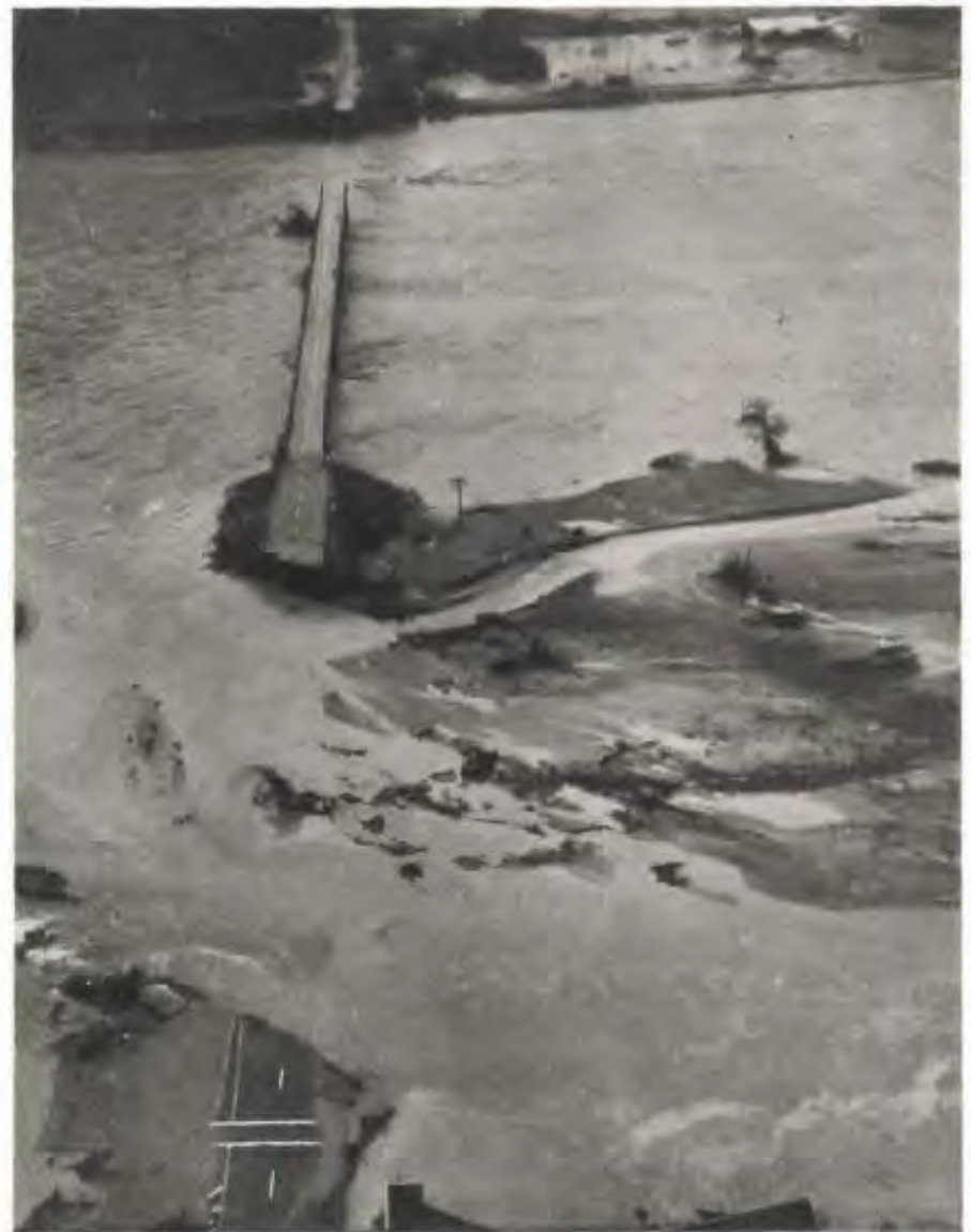
FIGURE 22.—Main Street, Klamath, Calif., after flood of December 23, 1964. Klamath River floodflows destroyed the town and damaged U.S. Highway 101 and the Douglas Memorial Bridge. Photograph by Eureka Newspapers, Inc.
