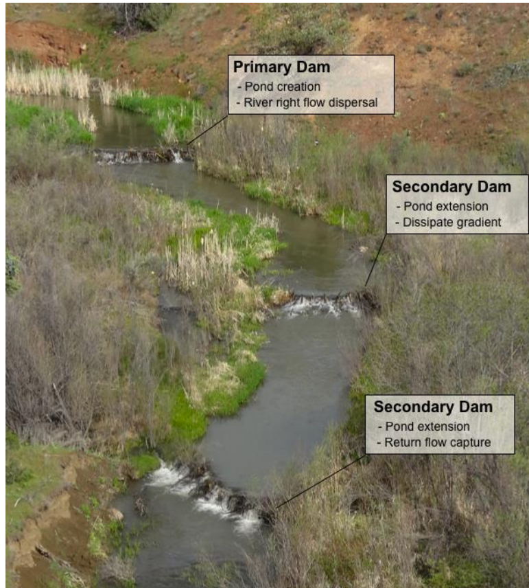
Figure 16 - Structure complex on Bridge Creek, OR. A starter dam is shown at the top of photo which has led to ponding upstream and downstream flow over the floodplain. Two secondary dams are shown downstream, extending the length of the ponded area and encouraging additional flow onto the RR floodplain. Not visible in the photo is a high-flow side channel on RL that is now regularly inundated due to ponding from the upstream secondary dam pictured in the middle of the photo. (Figure from Weber et al., (2015))
