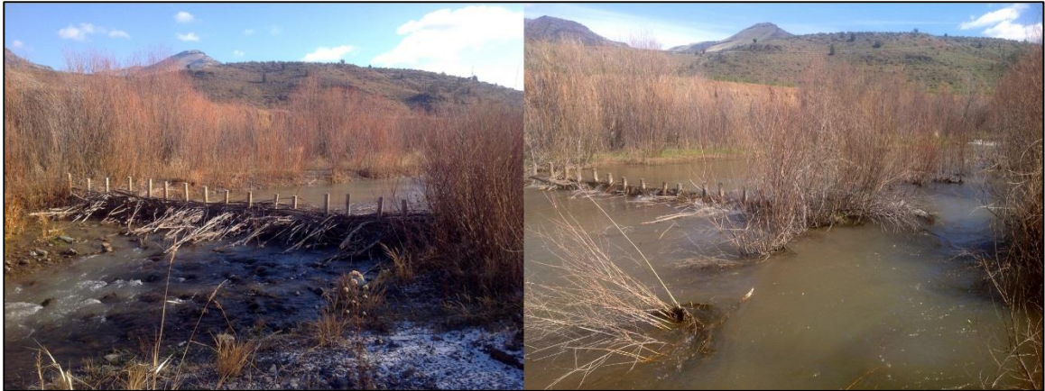
Figure 18 - Example of a primary dam on Bridge Creek, OR after construction (left panel) and extensive flooding onto adjacent floodplain surfaces the following spring (right panel). Source: Nick Weber.
