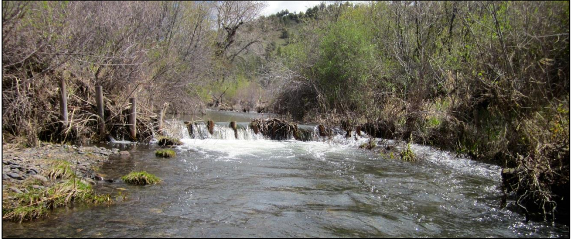
Figure 19 - Example of primary dam structure installed by the Oregon Department of Fish and Wildlife in 2012 on Beach Creek in the Upper Mainstem John Day River. Structures were designed to support greater habitat complexity and increase water storage during low base flow conditions. Source: Nick Weber
