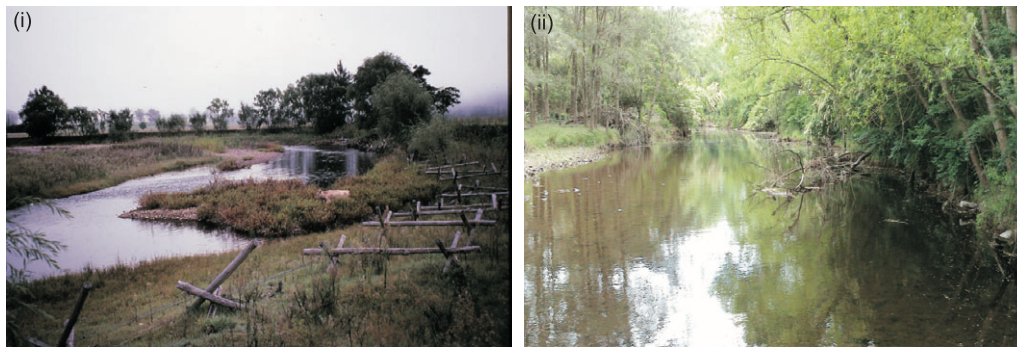
(b) Reinstatement of a wandering gravel bed river via wood installation and revegetation
