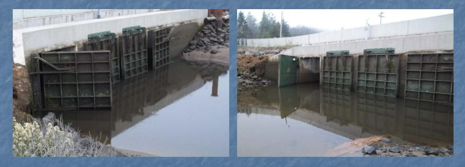
Top Hinge Side Hinge Array with MTR
