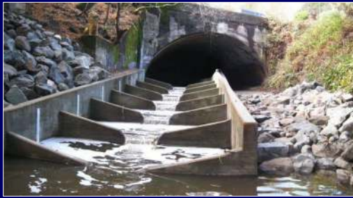
Partial Width Pool-and-Chute Fishway
