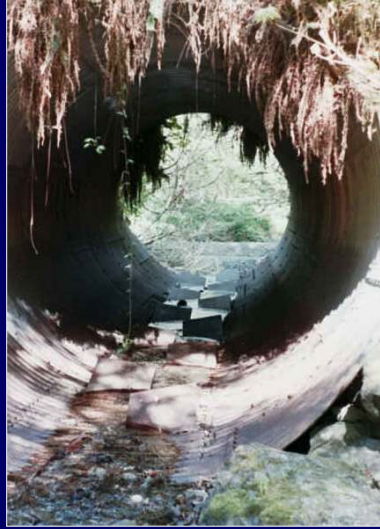
Lack of Depth at Low Flows Functional over Narrow Flow Range
