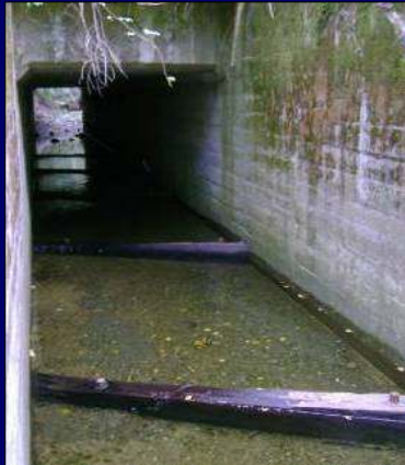
Wooden Angle Baffle (looking downstream)
