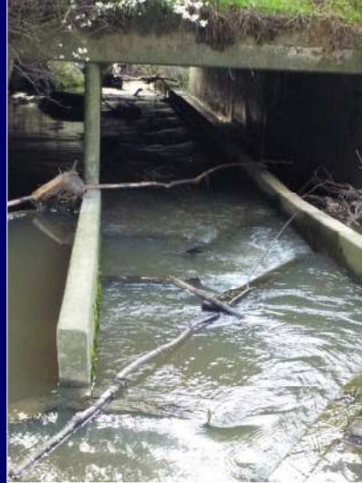
Tend to Catch Debris!!! Slot Velocities too Fast for Small Fish
