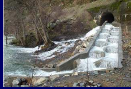
Bypass "Serpentine" Pool-and-Weir
