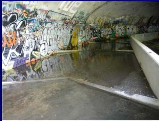
Double Angle Baffles for Wide Culvert ("Vortex Baffle") (looking upstream)
