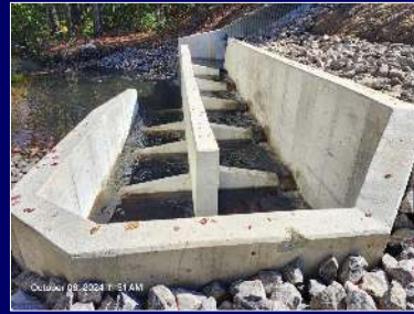
Bypass Pool-and-Weir Fishway
