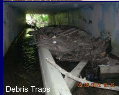
Invert Paving with steel Corner Baffles Added
