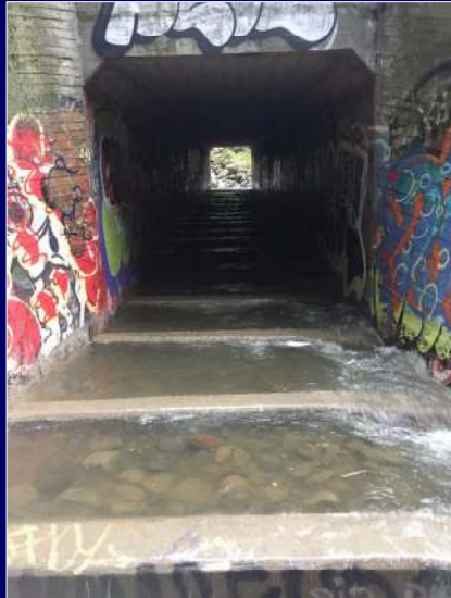
Concrete Angled Baffle Retrofit
