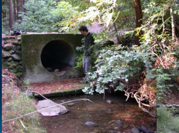
Outlet Headwall and Apron
