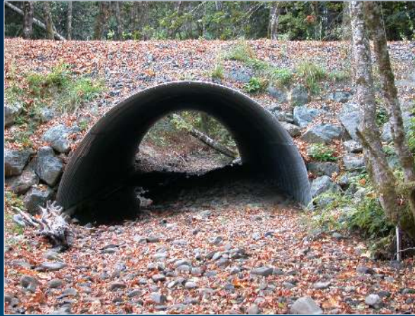
Sullivan Gulch Stream Simulation Culvert Replacement
