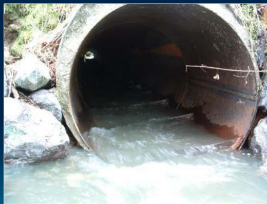
Corner Baffles in Slipped Line Culvert
