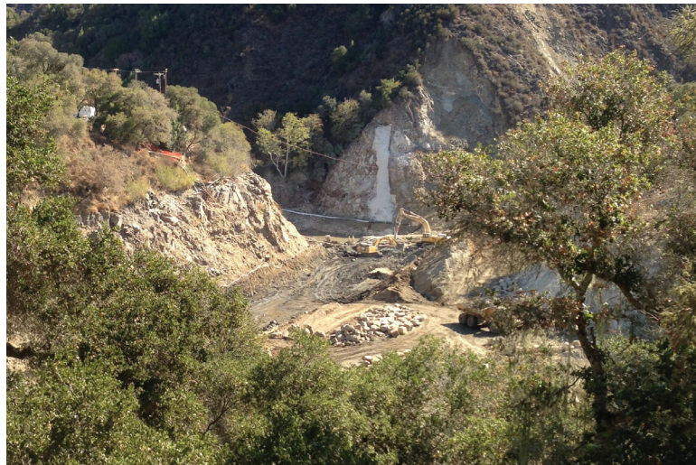
Remnants of San Clemente dam after dam removal.
