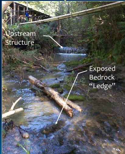
Upstream of perched culvert, prior to removal
