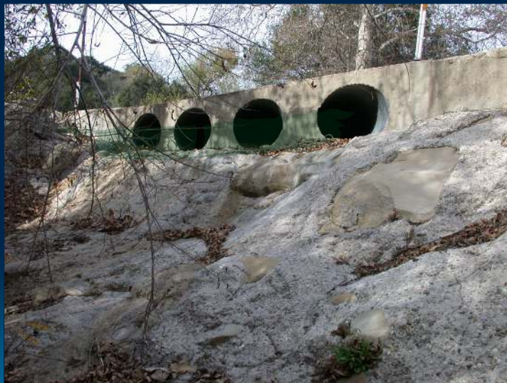
Vented low-water crossing (ford) with 8.7 feet of drop.
