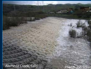
Alameda Creek, Calif. Photo: Jon Stead Armored Utility Crossings
