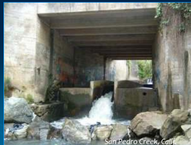
San Pedro Creek, Calif. Perched Fishway Entrances
