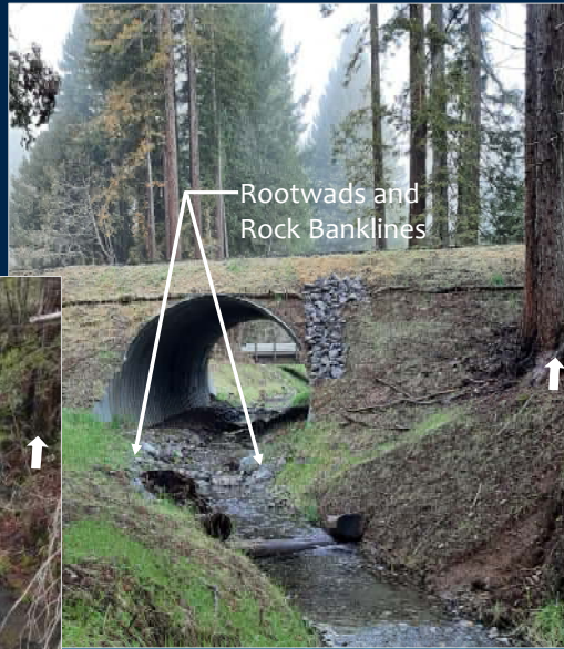
After - Restored Streambanks at Outlet
