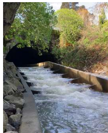
San Anselmo Creek Fish Ladder, Marin, CA
