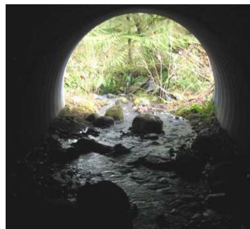
Image from CDFW Part XII (2009), Stossel Creek culvert
