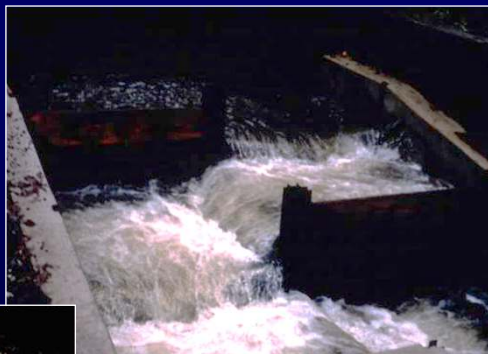
Fish passage design flow (for Pacific salmon) EDF = 4 ft-lb/sec/ft 3
