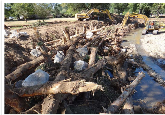
Combination of native streambank material, boulders, and logs used as ballast.
