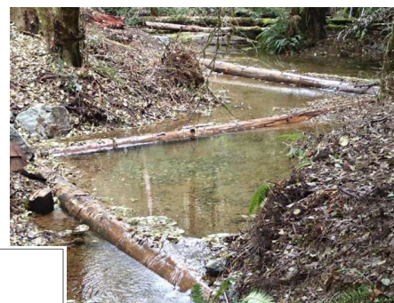
Diagonal log weirs in series. Photo credit: Sanctuary Forest.
