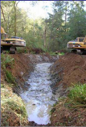
1. Grading and Compact Subgrade
