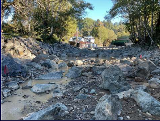
Rowdy Creek Fish Hatchery - Incised Channel below US101 Chutes and Pools Roughened Channel 5 Chutes and Pools | Total Fall = 10 feet
