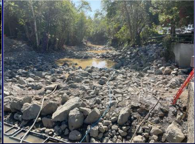
Rowdy Creek Fish Hatchery - Incised Channel below US101 Chutes and Pools Roughened Channel 5 Chutes and Pools | Total Fall = 10 feet
