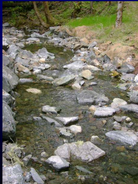
Grub Creek "Rock Ramp"
