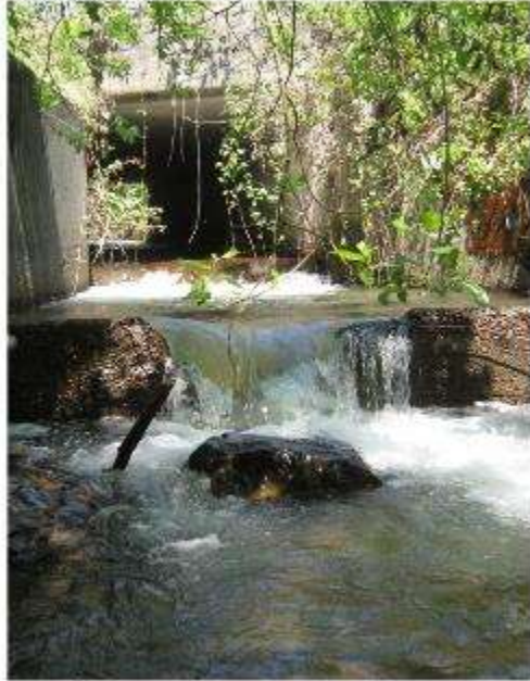
Pre-treatment: Before Replacement. Drop at culvert outlet. Photo taken on and courtesy of Caltrans.
